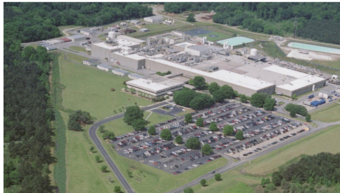
Westinghouse Columbia Fuel Fabrication Facility Site
