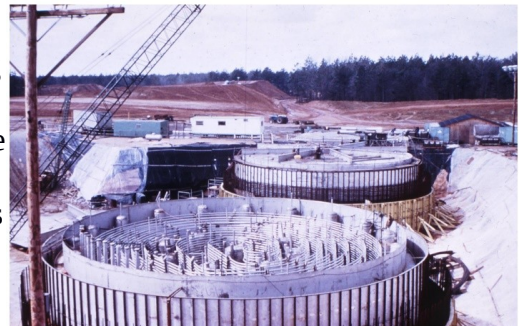
Fig 6 HLW tanks during construction [1]
